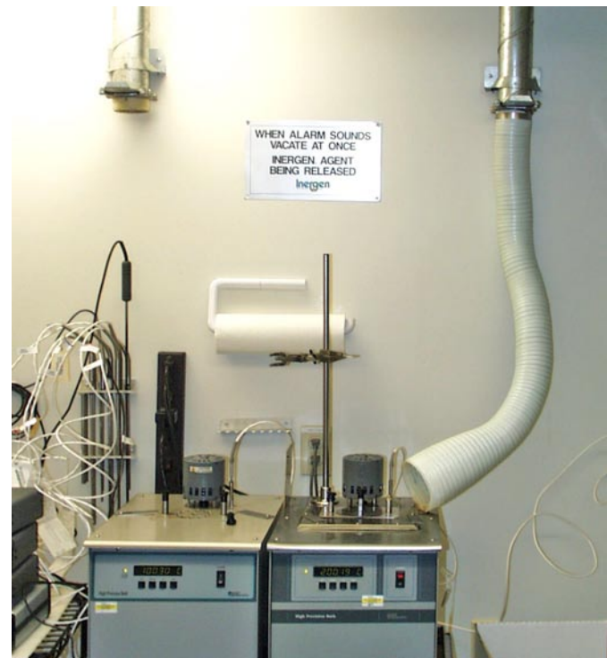
Figure 1 Ventilation system for removing oil vapors.
